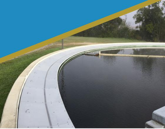
Several factors can influence a clarifier’s performance at a waste water treatment facility. One of the toughest issues is the build-up of algae along the effluent launder channel. Excessive algae growth can limit the flow along the channel and reduce the clarifier’s effectiveness. It is also a chronic maintenance issue that requires frequent cleaning. Failure to perform these cleanings affects the overall productivity of the facility.
